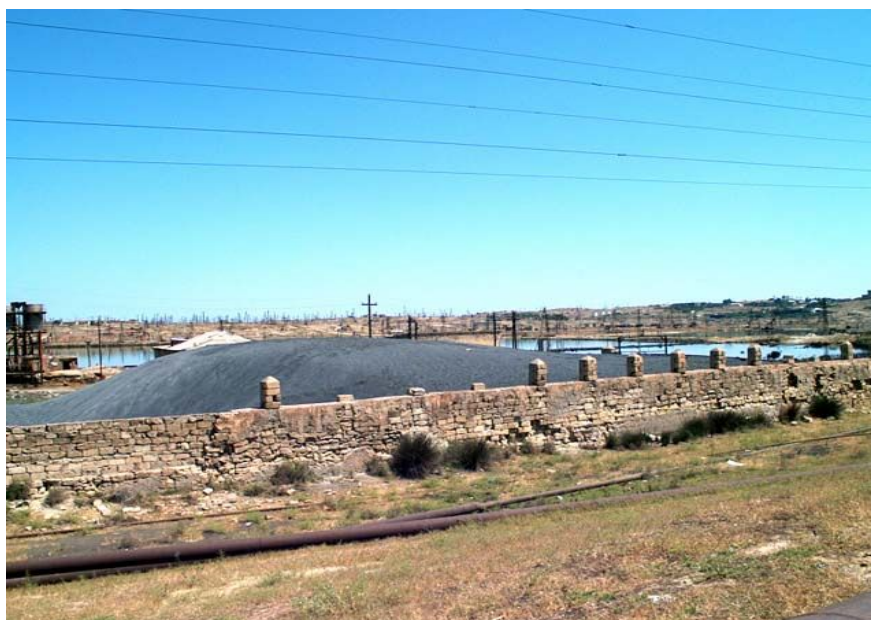
Fig. 4. Environmental contamination by iodine plants. On the left – accumulations of high-radioactive activated coal.
