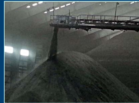
Coal yard (interior)
