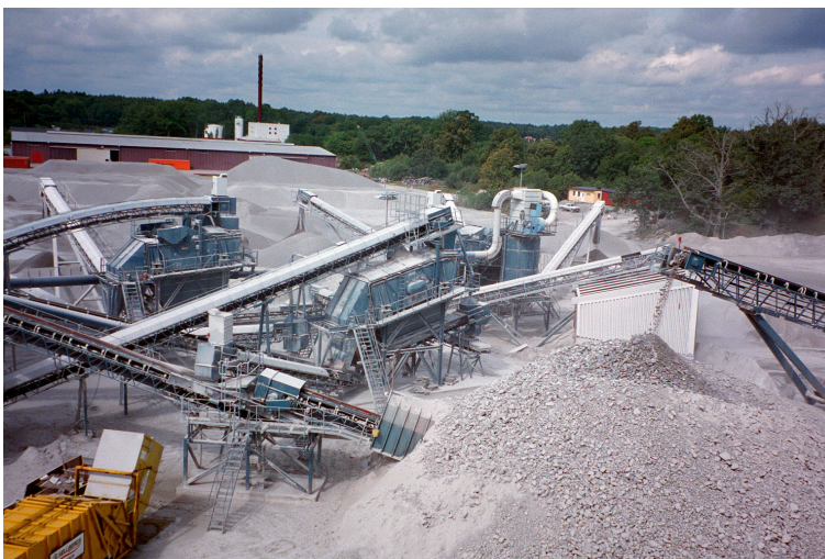
Figure 3. Crushing plant at the Blekinge Coast Gneiss quarry.
