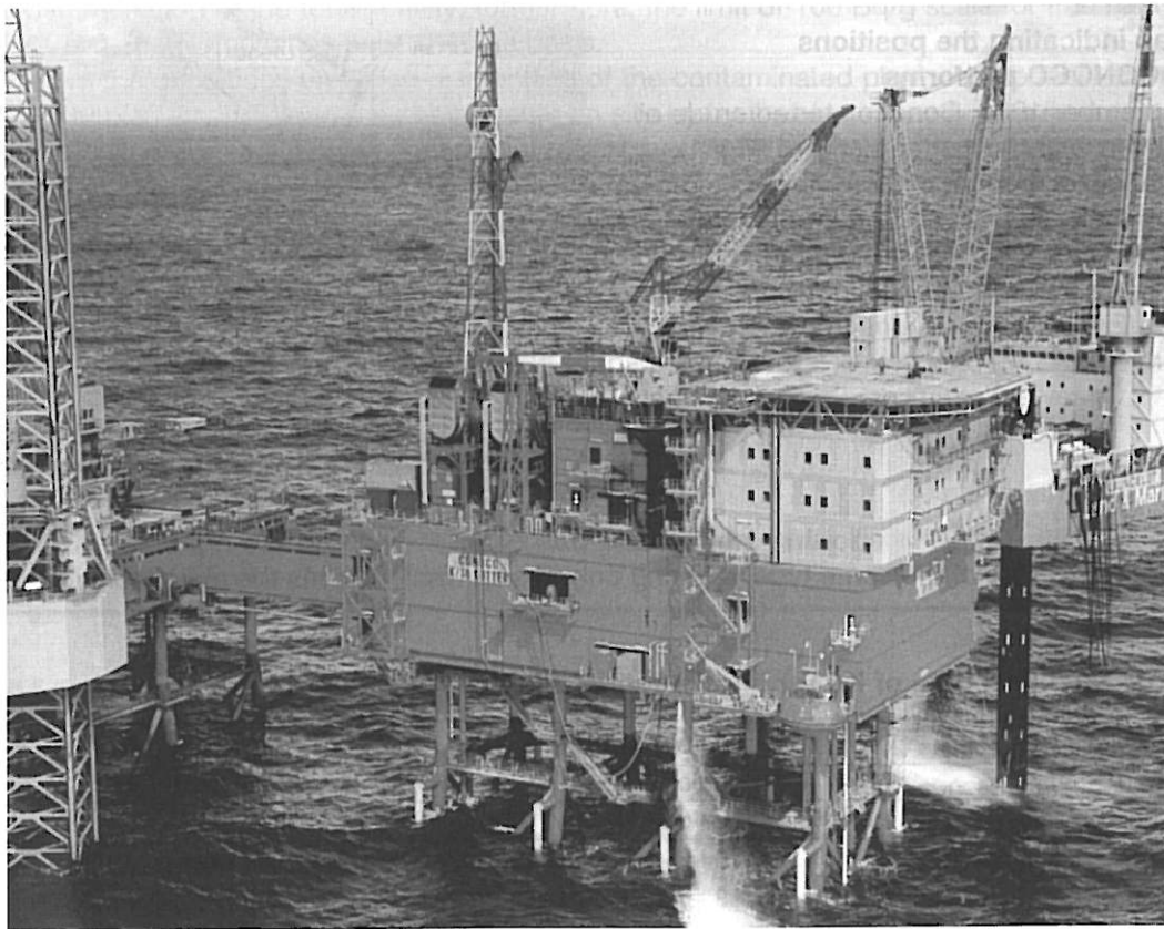
Fig. 1: Oil platform Kotter
