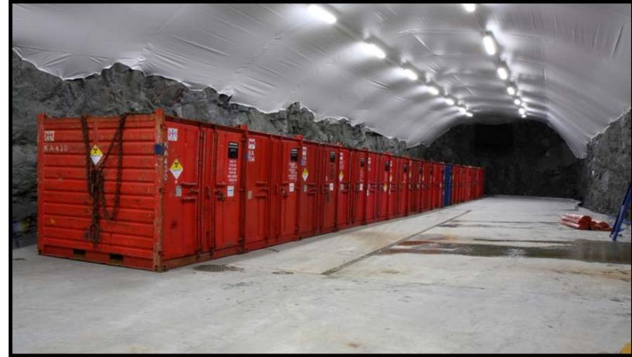
**Containers with NORM drums are received at quayside and transported unopened to the Storage & Conditioning Tunnel.**
