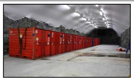
Containers with NORM drums are received at quayside and transported unopened to the Storage & Conditioning Tunnel.
