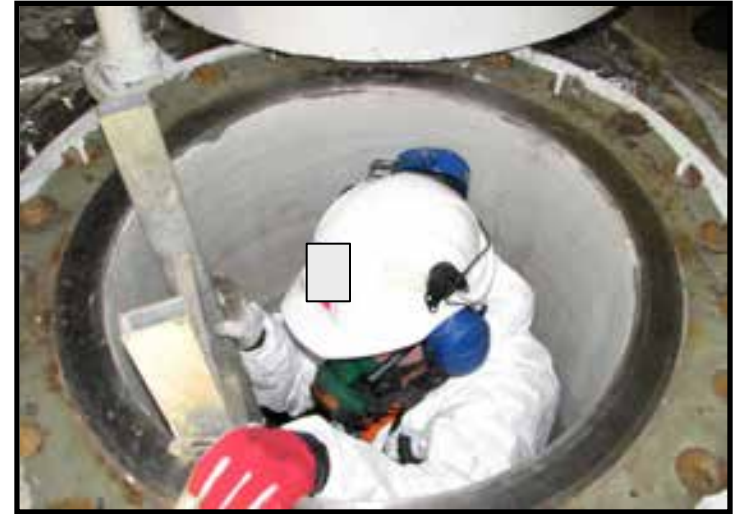
Separator tank entry (observe the scaling)
