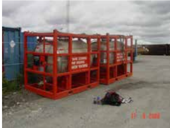
Tanks with NORM contaminated sludge
