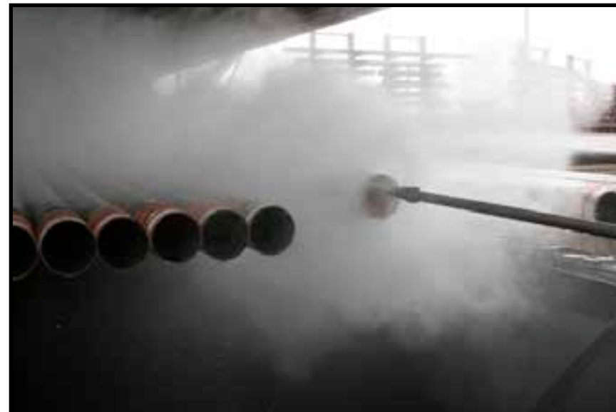
Water jetting at 2 000 – 3 000 bars
