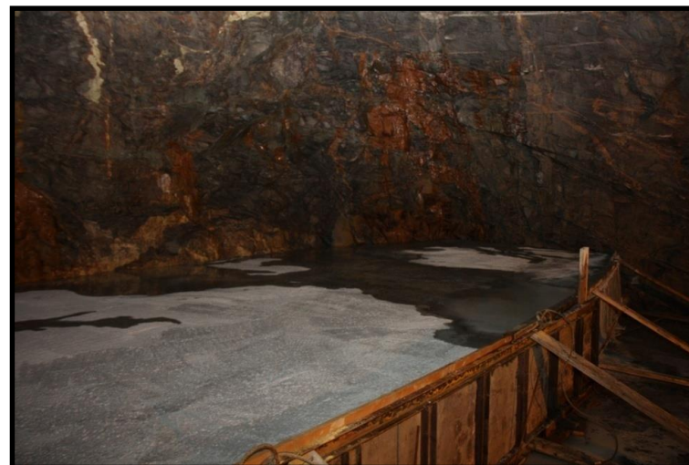
First shipment drums grouted and secured.
