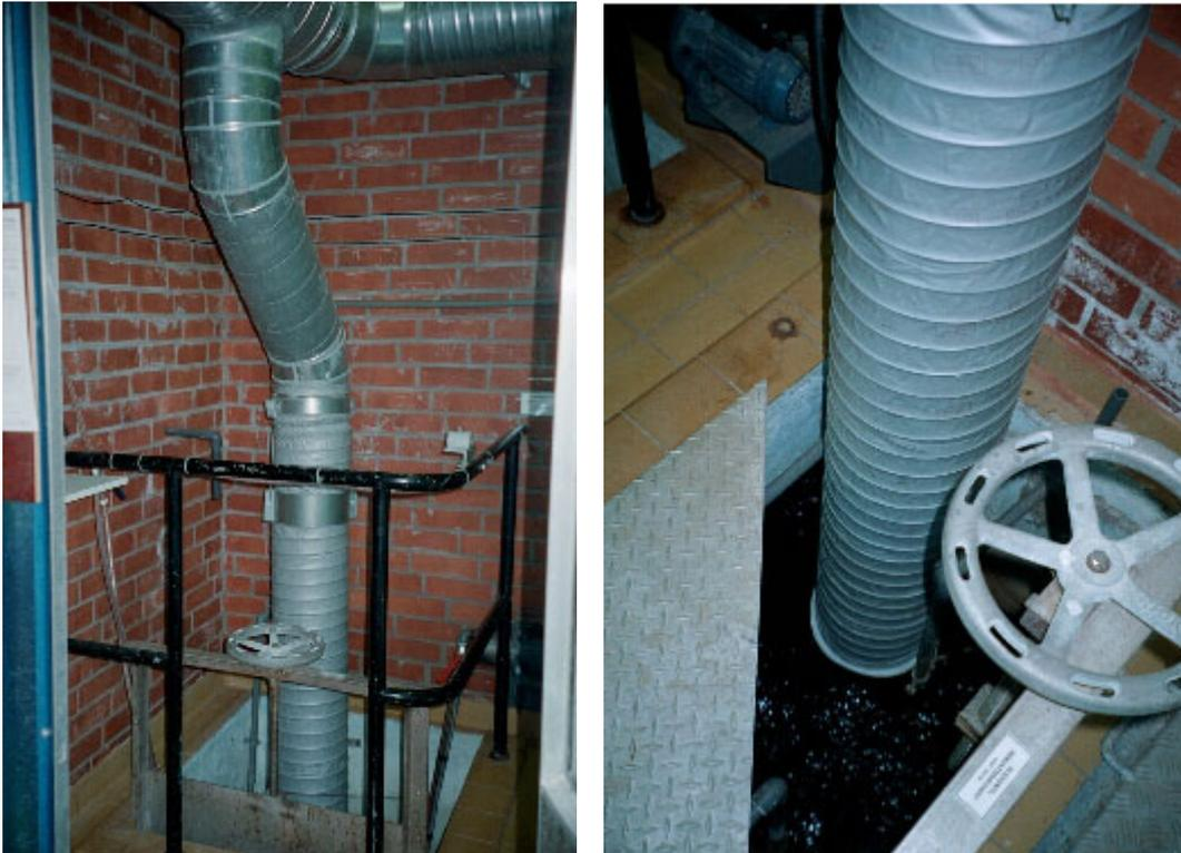
Fig.3: Inspection opening to the mixing chamber
