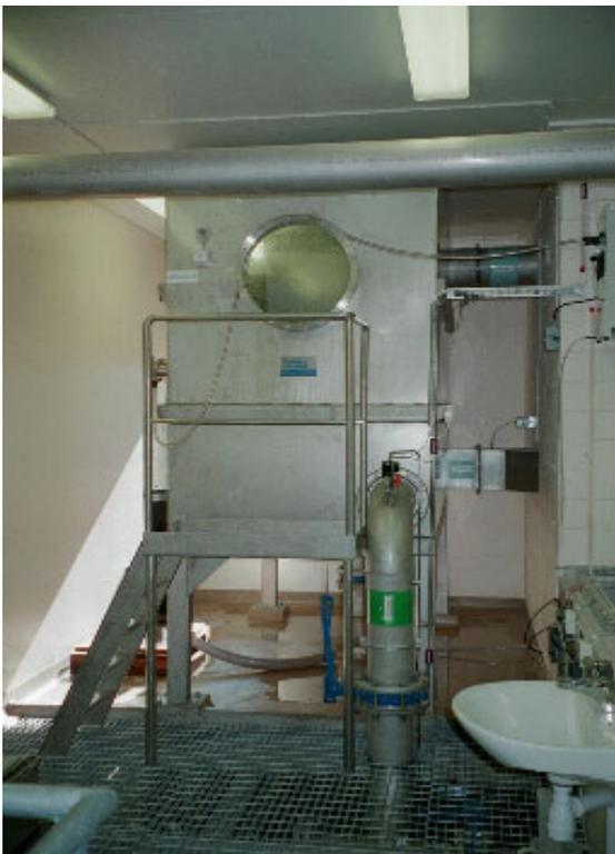
Fig.7: Equipment for intense aeration of the water at the Kolbäck waterworks
